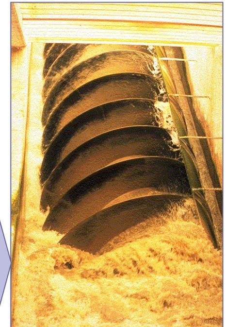
Archimedes's water screw in its modern form, as implemented in the wastewater treatment plant of Athens (1 of 5 screws that pump 1 million m<sup>3</sup> per day).
