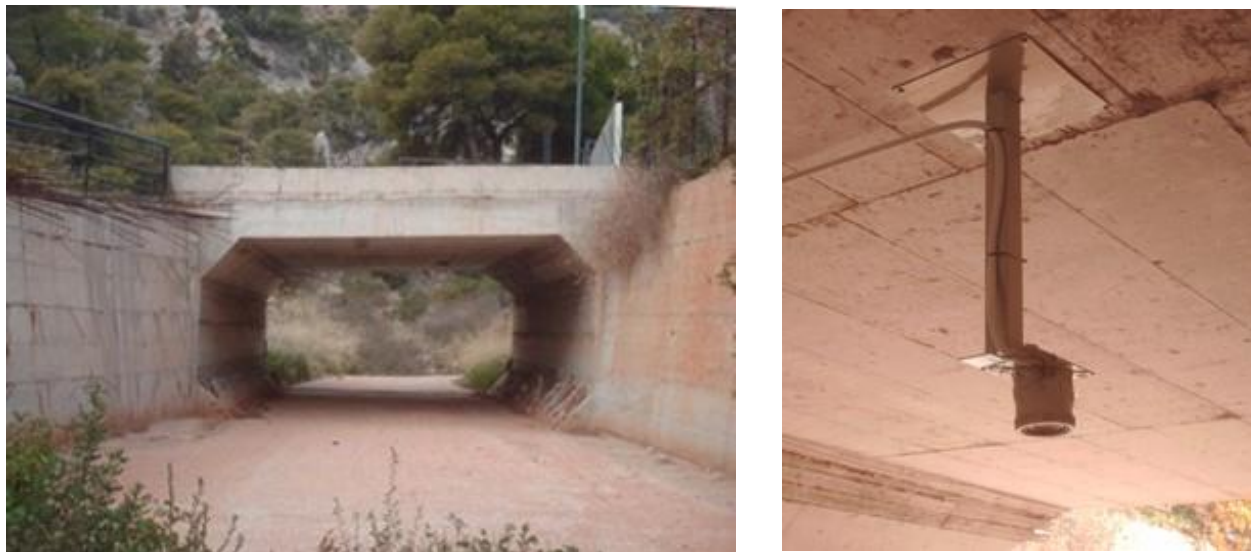
Picture 4.3. Culvert cross-section (left) and stage-gauging sensor (right) (Koussis et al. , 2012)
