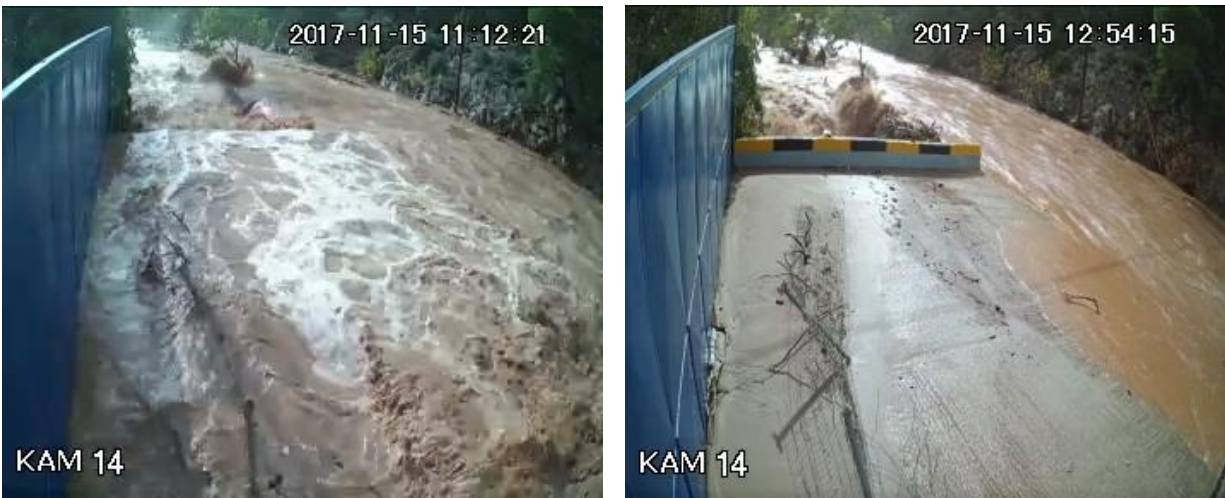
Picture 6.1. CCTV footage of the culvert during the flood
