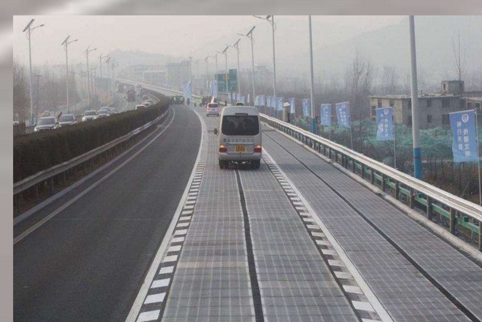
Fig.7. The first solar-powered highway in China.
