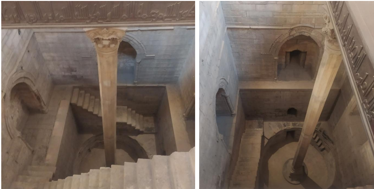
Figure 1.11 The Roda Nilometer, near Cairo. Water entered through three tunnels and filled the Nilometer chamber up to river level. The measurements were taken on the marble octagonal column (with a Corinthian crown) standing in the centre of the chamber; the column is graded and divided into 19 cubits (each slightly more than 0.5 m) and could measure floods up to about 9.2 m. A maximum level below the 16 th mark could portend drought and famine and a level above the 19 th mark meant catastrophic flood. (Photos courtesy of Nikos Mamassis.)
