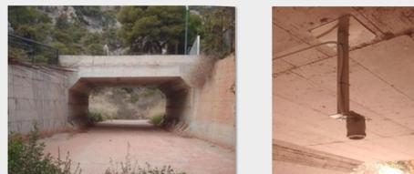
Cross-section of the culvert (left) and the automatic stage recorder (right)
