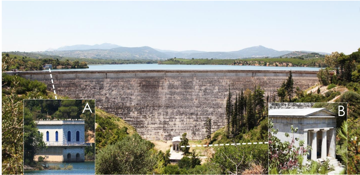
Figure 7. Example of architecturally designed dam (Marathon dam in Greece). Picture of the downstream face of the dam, which is overlaid with marble from the mine of Penteli that was also used to build the Temple of Parthenon, including pictures of architecturally designed appurtenant structures: (A) water intake tower, with similar design with the downstream face of the dam and (B) reservoir control building at the base of the dam, built to resemble the ancient temple built after the victorious battle of Marathon (480 BCE) and symbolizing the victory of modern Athens in the battle against water scarcity. The dam of Marathon is not a hydroelectric dam but is indicative of the architectural adaptability of dams and their appurtenant structures, that can, and has been utilized in hundreds of hydroelectric dams internationally. Technical information on Marathon dam can be found in Soulis et al. [175].
