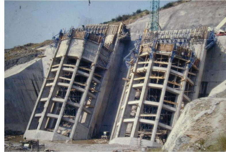
**Stratos dam: inclined intakes under construction**
