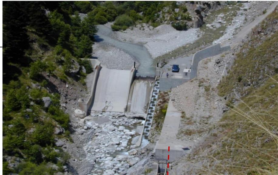
Spillway - water intake - fish ladder
