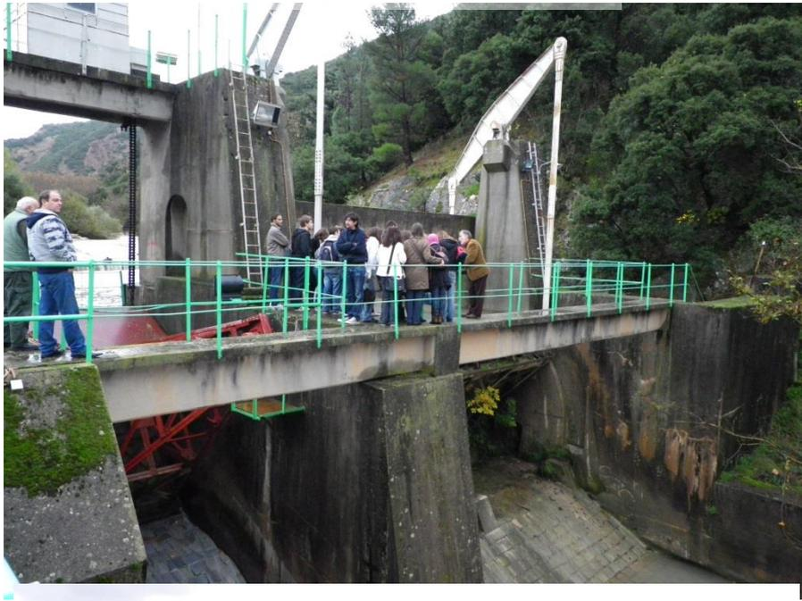
**Sand trap – desilter – sedimentation tank**
