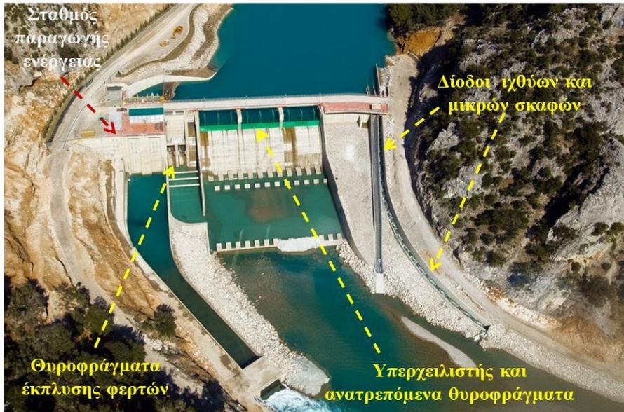
2 turbines Kaplan S-Type, power 5.93 MW (5-40 m<sup>3</sup>/s)
