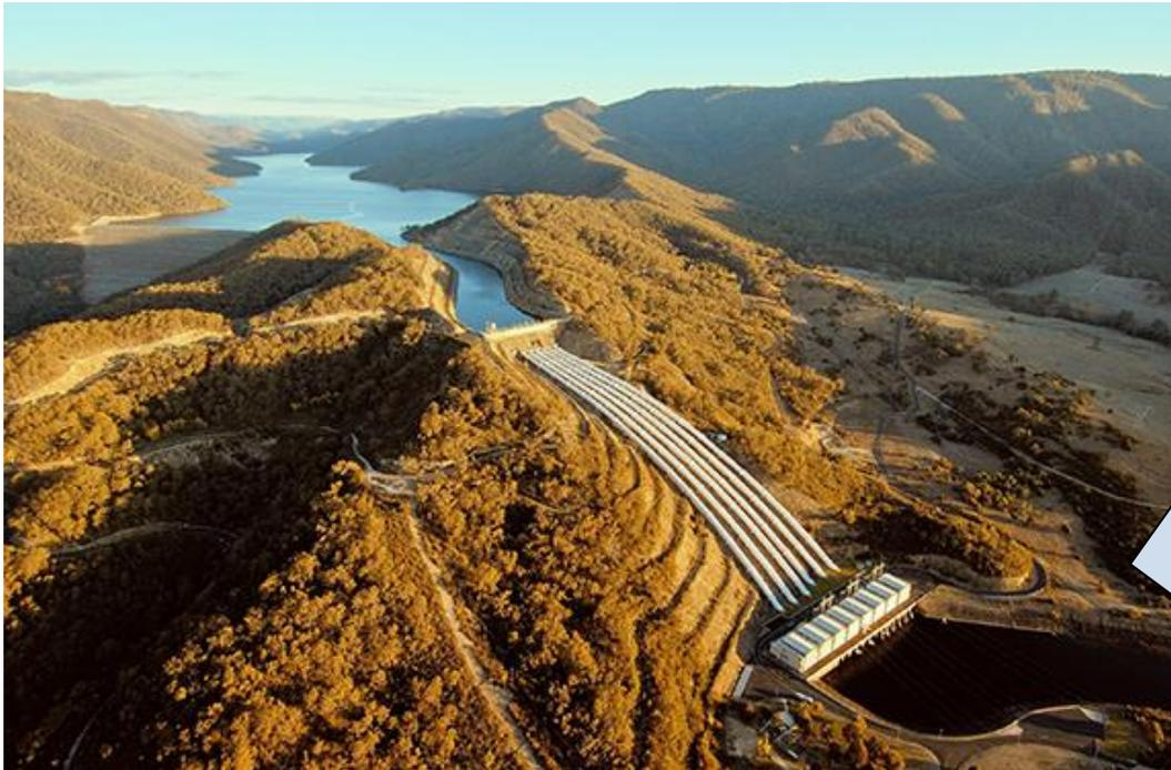
**Tumut 3:** First major pumped-storage station in Australia (constructed in 1968, entered into operation in 1972, upgraded in 2012); six turbines of combined power capacity of 1800 MW, three of them also operate as pumps; rated head 150.9 m; six pipelines of 488 m length and 5.6 m diameter; lower storage element: Talbingo reservoir (920 hm<sup>3</sup>), upper element: Jounama reservoir (43.5 hm<sup>3</sup>)
