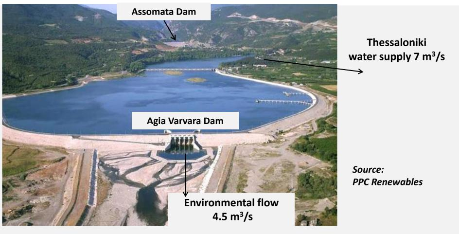
It is constructed at the foot of the Agia Varvara regulatory dam. The SHPP belongs to the Public Power Corporation (PPC) and exploits the environmental flow of Aliakmon river. It includes a Kaplan S-type horizontal-axis turbine of 23 m head and 0.92 MW capacity. It operates from 2008 and has mean annual electrical energy production of 4.5 GWh.
