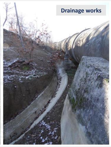
Diversion penstock of Plastiras hydropower system: length 2985 m, diameter ranging from 2.60 to 3.50 m, elevation difference ~570 m
