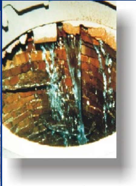
Manhole improperly covered
