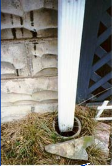
Illegal connection roof drainage into sewer system
