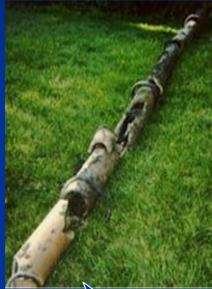
Eroded sewer pipe
