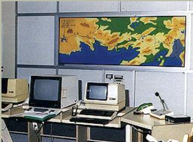
Aqueduct supervising & control centre
