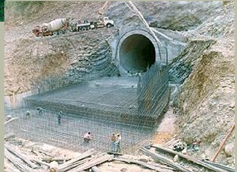
Construction of the Evinos-Mornos connection tunnel →
