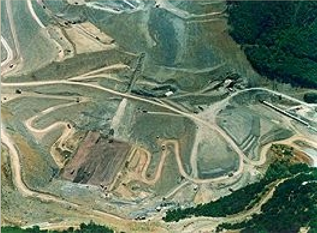
← Evinos dam during construction
