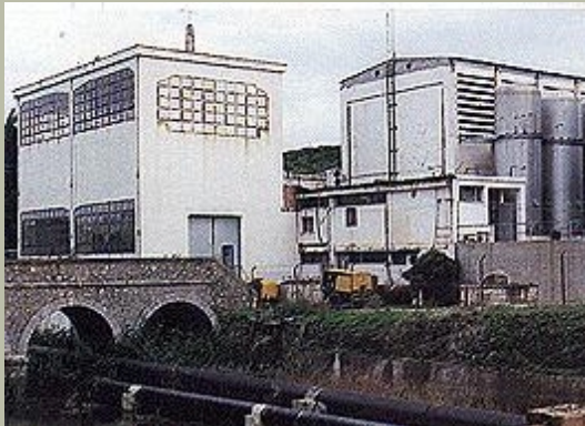
Yliki, main pumping station
