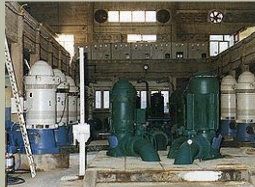
Kiourka pumping station
